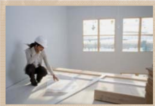
Business building renovation
