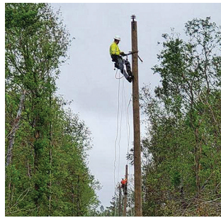
The crews work to string line.
