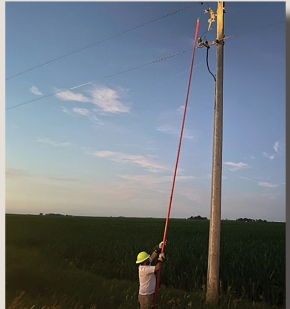
Lineman Andrew Stupka restores a power outage.
